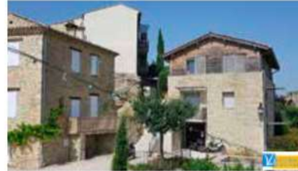
La Tour, Faucon, Mistral Habitat F. Chabert, C. Mendez, architectes
